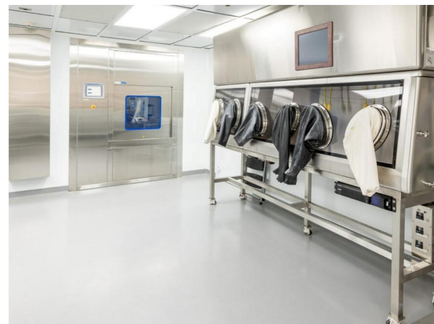
↑ Figure 3: Example of an isolator in a cleanroom space
